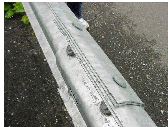
TYPICAL NESTED PANEL MID-SPAN SPLICE
