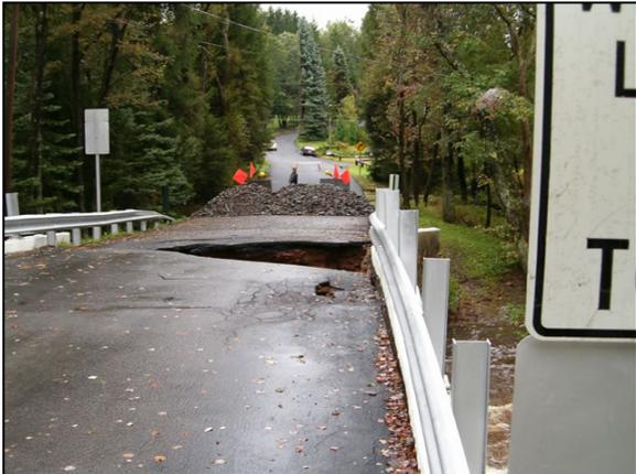
**Extreme settlement damage in the roadway, causing a hole in the roadway behind the bridge abutments**
