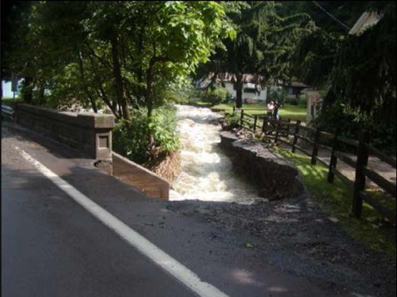
**Embankment erosion damage under the adjacent roadway. The roadway shoulder has fallen away**
