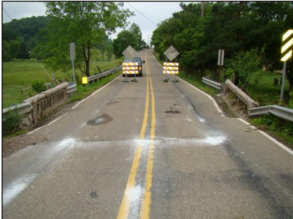
**Settlement damage in the roadway due to settlement and tilt of the bridge abutment in the picture to the right**
