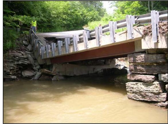
**Extreme settlement damage in the abutment**
