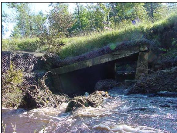
**Settlement damage in the abutment due to scour underneath the bridge abutment**
