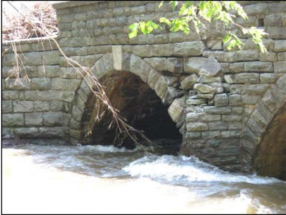
**Settlement damage in the stone masonry pier and some collapsing in the arch**
