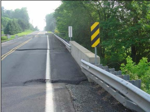
**Settlement damage in the approach fill behind the abutments as viewed from the roadway above the bridge.**
