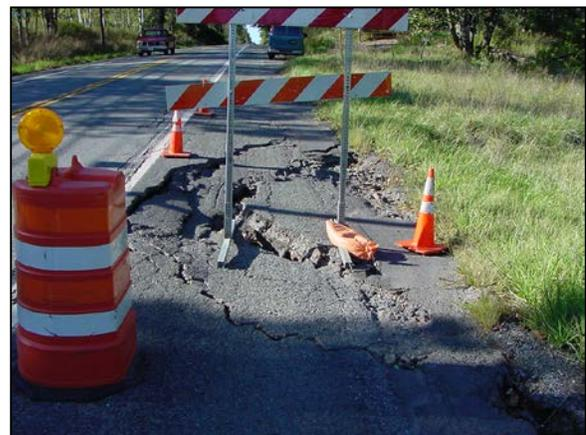
**Settlement damage effect on the roadway due to scour underneath the bridge abutment in the picture to the left**
