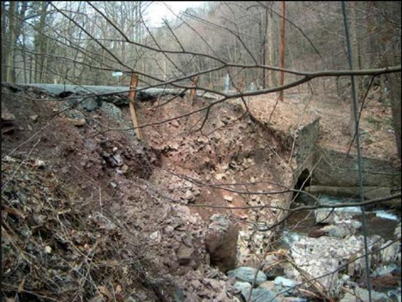
**Embankment erosion damage and part of bridge has collapsed into the stream channel**
