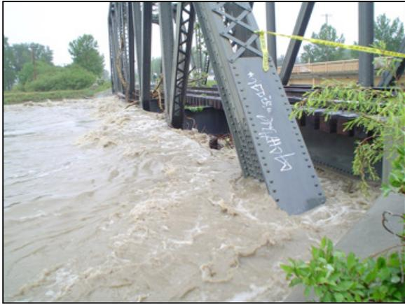
**Pressure flow – water is flowing against or the bridge superstructure. Water levels may continue to rise and flow over the bridge; this is called “overtopping”.**
