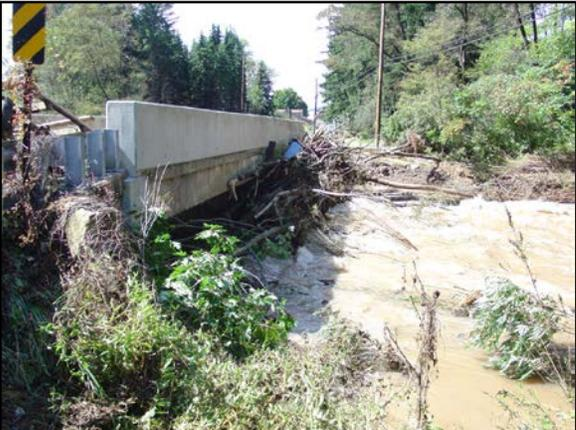
**Severe debris buildup of tree branches, caught against the bridge blocking more than 25% of the span opening**
