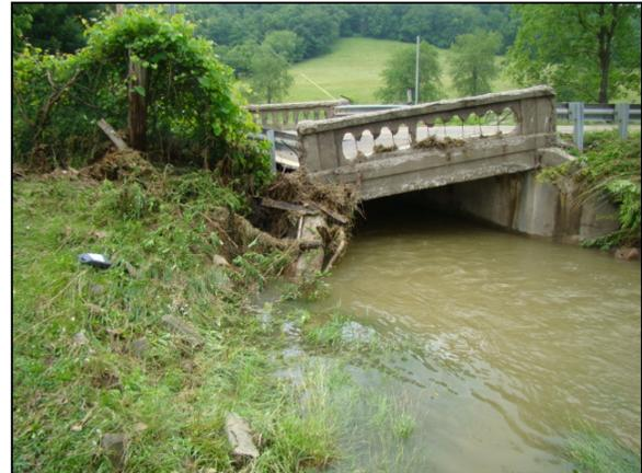
**Settlement damage of the bridge causing tilt and roadway settlement damage in the picture to the left**
