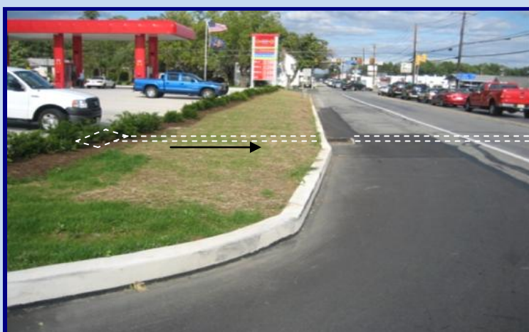
Figure 1.3.2- Site storm water directed into PennDOT Right-of-Way through enclosed surface storm water facilities tied into an existing inlet which is part of a larger drainage system.
