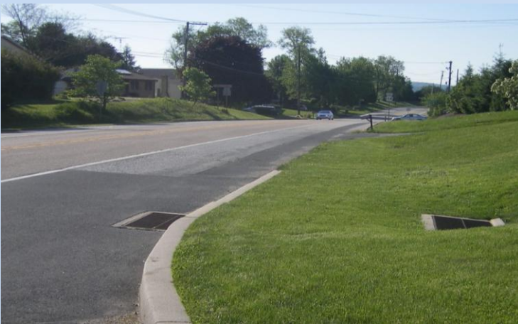
Figure 2.1.1- Conventional installation where enclosed surface pipe connect to highway drainage facility
